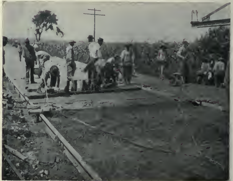
Fig. 4—Laying brick, Paris, Ill.
